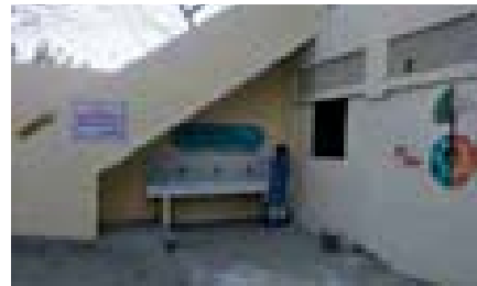
Renovated hand wash area
