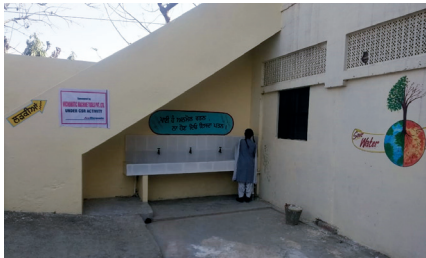
Renovated hand wash area
