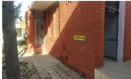
Cleaned and repainted washrooms
